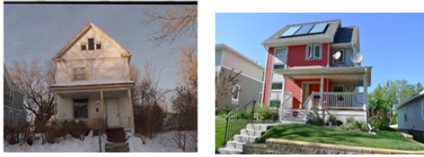
Habitat New Construction: Net Zero Home MHFA NSP3
